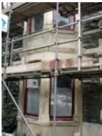
The Rainbow Centre behind scaffolding as we repaired the stonework and pointing during the summer break.
