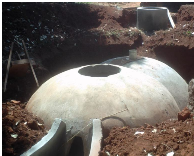
A biogas plant under construction in Bulindi Zone – Nabwigulu Sub County (2011).
