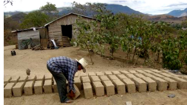
Stronger adobe brick homes will replace the temporary homes seen in the background.
