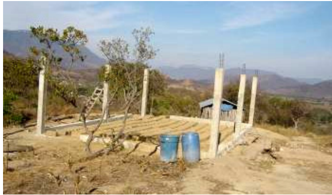
Work continues on the community center in San Pedrito
