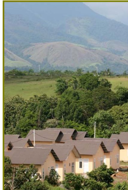
Nestled in the rolling hills of Jantho, Indonesia, is a new community of CARE-built homes. Construction workers are finishing the final installation of water and sanitation systems before the new owners can move in.
