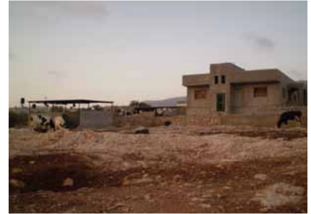
An unfinished Al Aqaba house and a shed for milk cows at left. Rebuilding Alliance will raise financing to complete the house.
