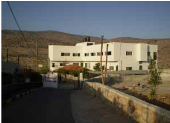
Al Aqaba's kindergarten, built by Rebuilding Alliance, has become a mixed-use building. Ground floor: the kindergarten and Mayor's office, 1st Floor: the Ibn Rush'd Library, classrooms, and Herbal Infusion Factory; 2nd Floor: Rural Women's Association's Sewing Cooperative.
