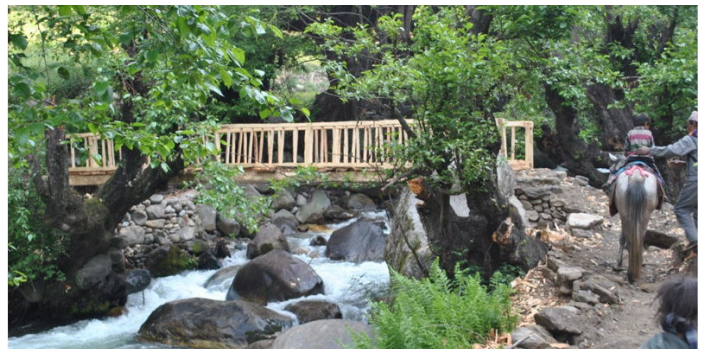
GHT Bridge Construction
