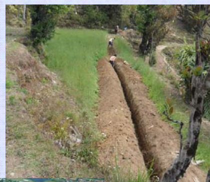
Above: Digging Trenches for a Water Project
