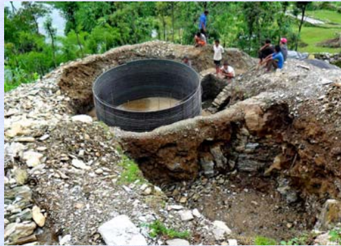
Above: Constructing water distribution tank
