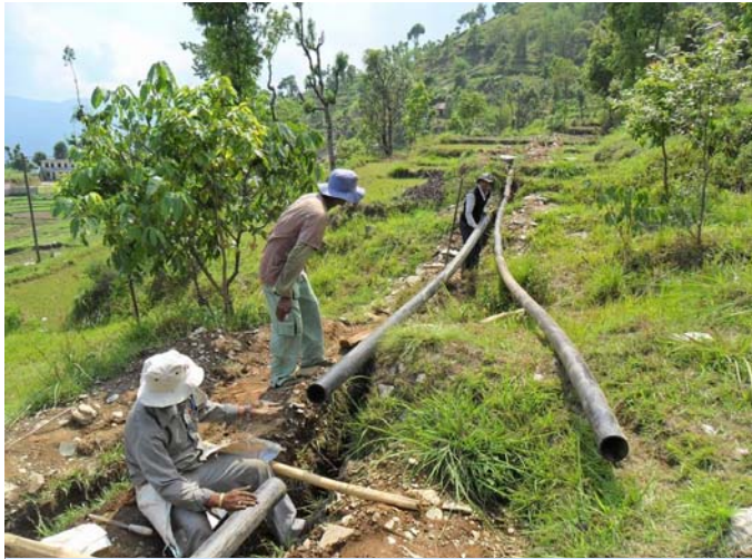
Laying the 40 km HDPE transmission line
