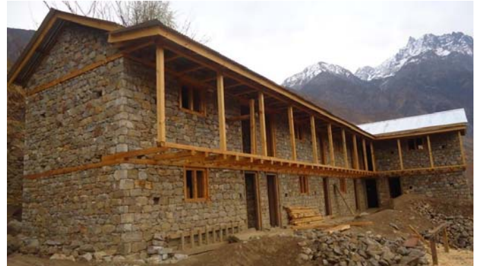
Thehe school construction
