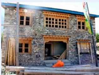
Muchu Gompa Restoration Project
