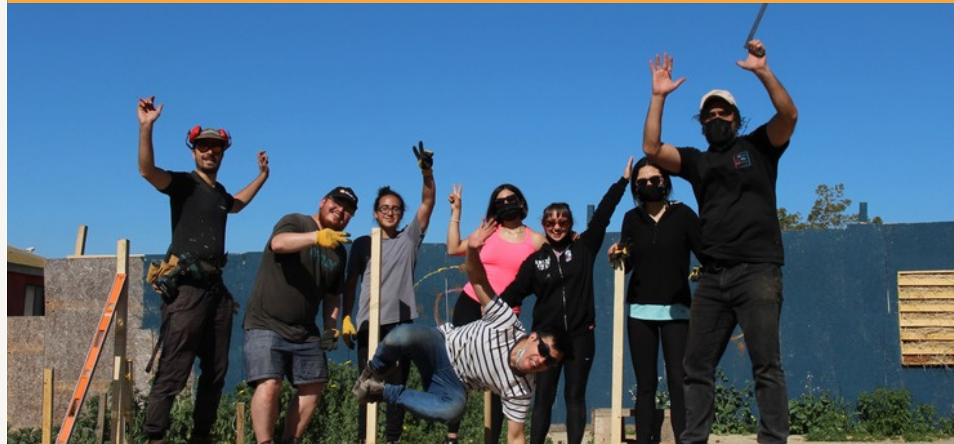
Greenhouse Construction, Ludoteca Concón
