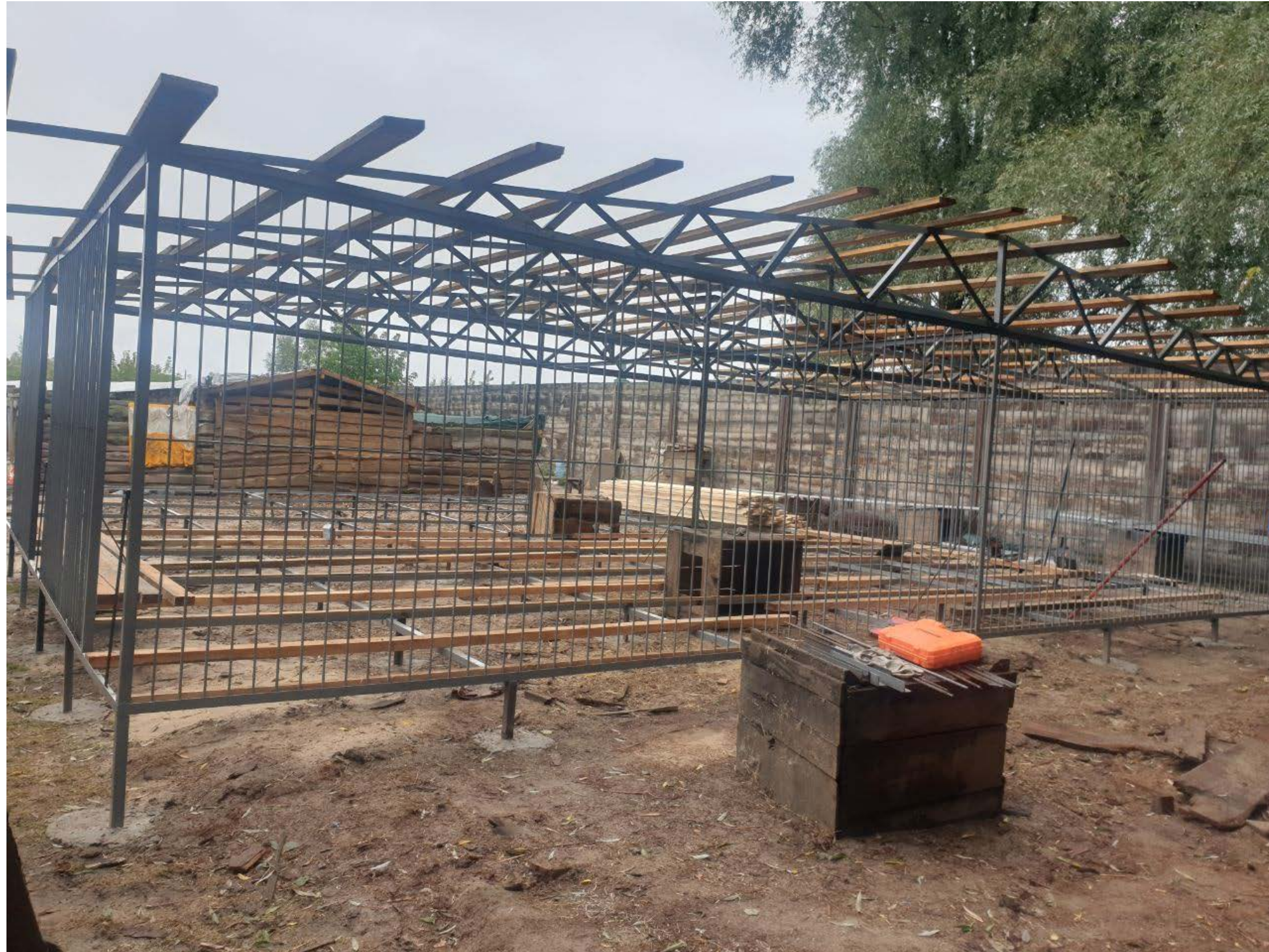
Building of the new modules.
