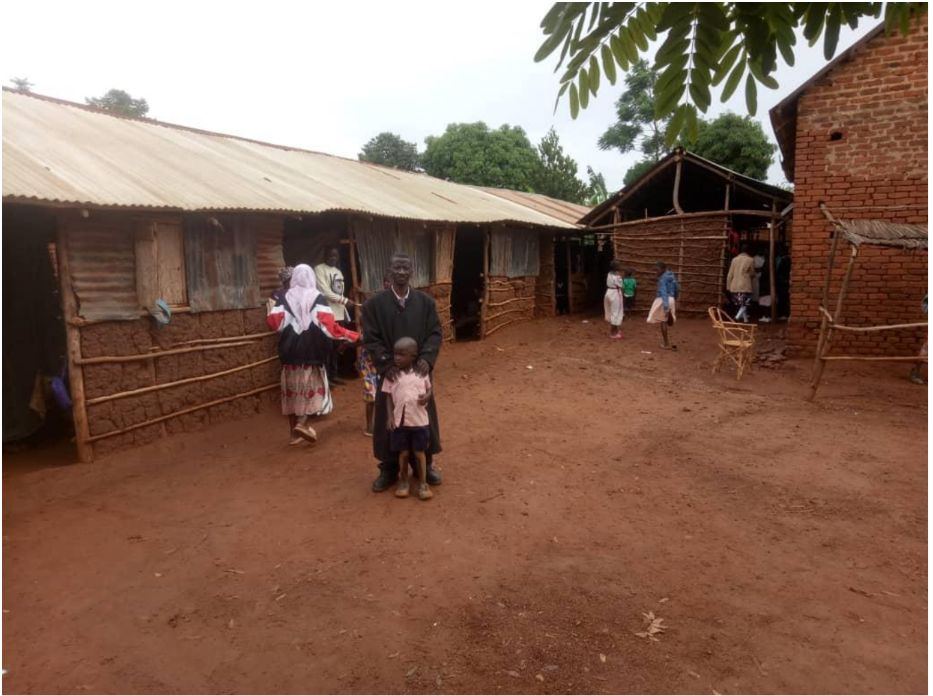
Figure 1: Crown Nursery and Primary School main block
