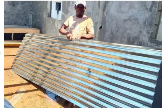
Above, rooftops were replaced with corrugated aluminum sheets.
