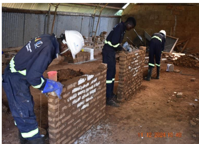
HCK training of the youths in brick laying and concrete practice at HCK vocational centre
