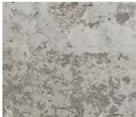
CONCRETE main structure frame
