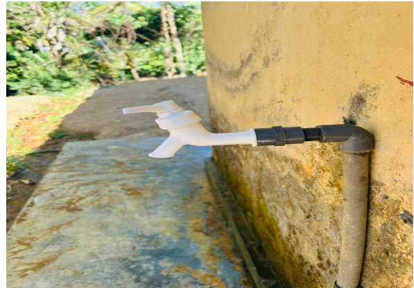
10. New tap and fitting after improvement
