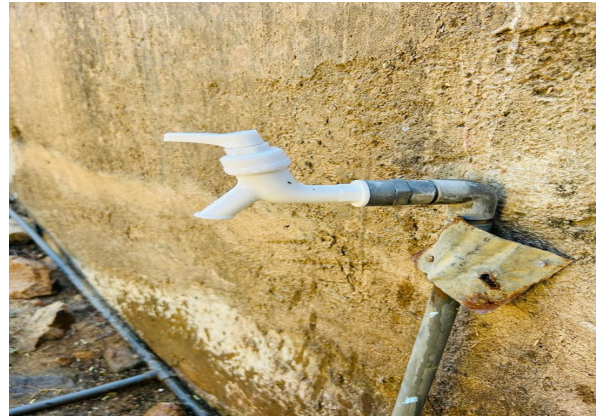
8. New external tap installed and functioning
