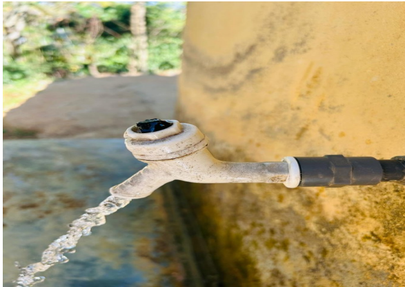
9. Existing tap and fitting before improvement
