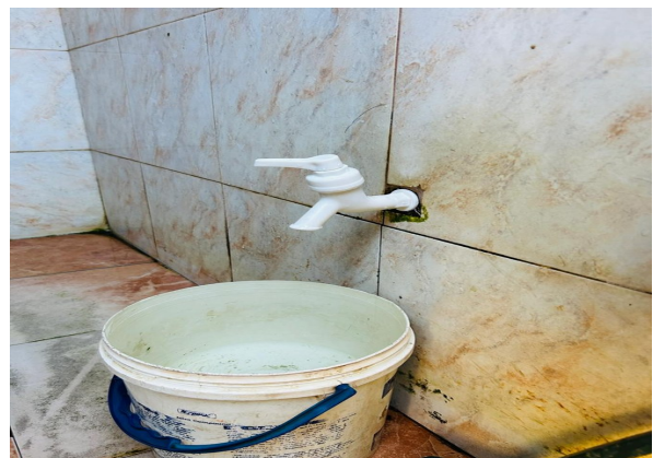
4. New washroom tap after replacement
