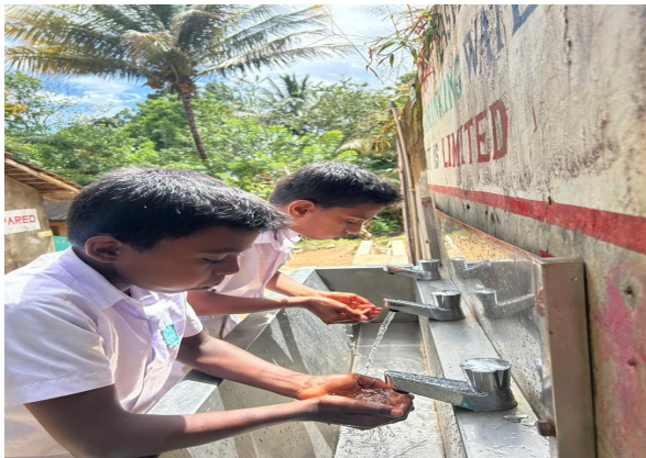
11. Students using the renovated handwashing facility
