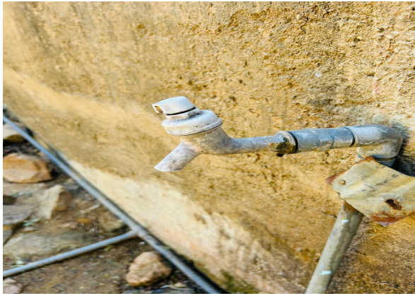
7. Existing external water tap before replacement
