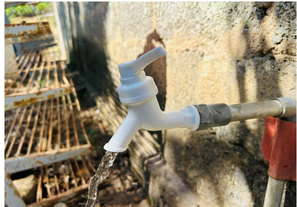
2. New tap installed at an improved water access point
