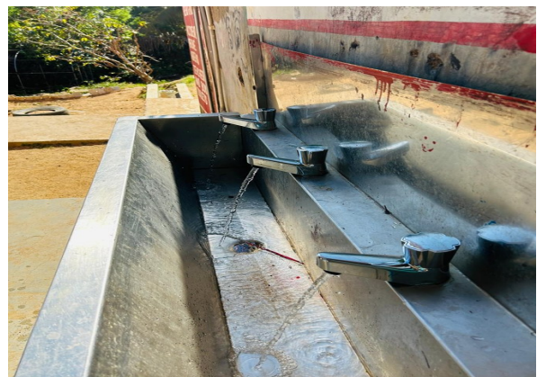
6. Renovated handwashing facility with new taps
