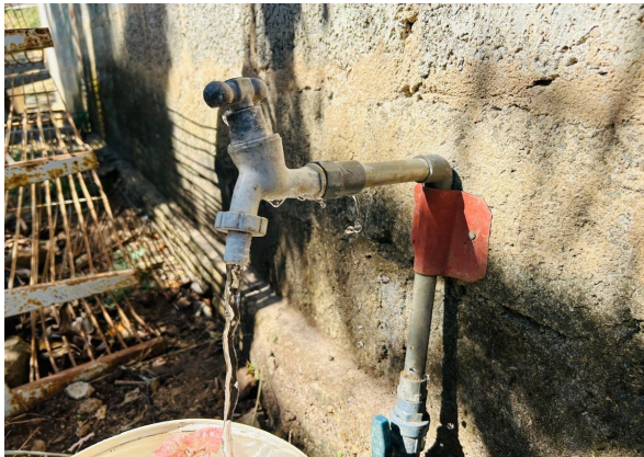
1. Existing water tap before improvement
