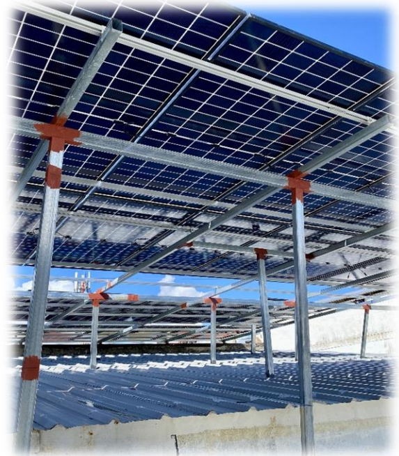
First phase of installation.
