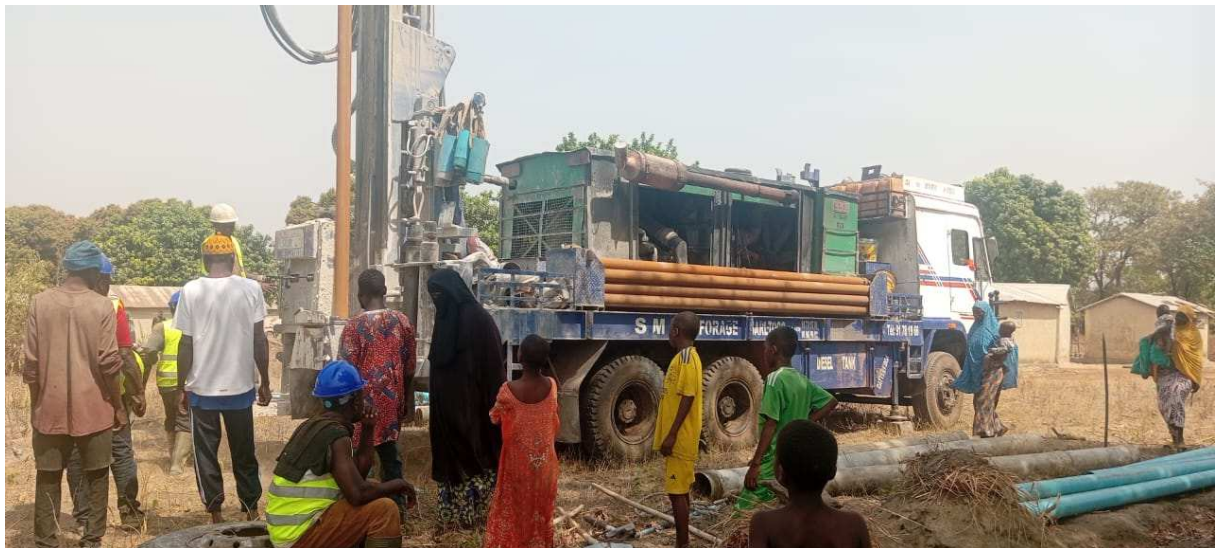
Well drilling at the Nigbaoudè village site on January 24, 2026
