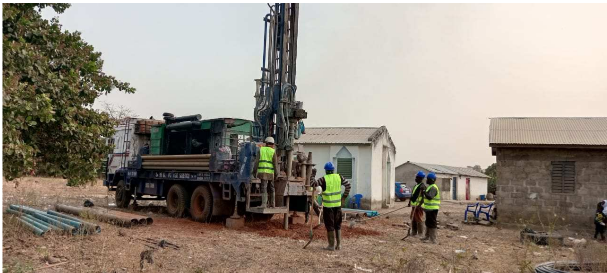
Well drilling at the site of Yéliwa village on January 21, 2026
