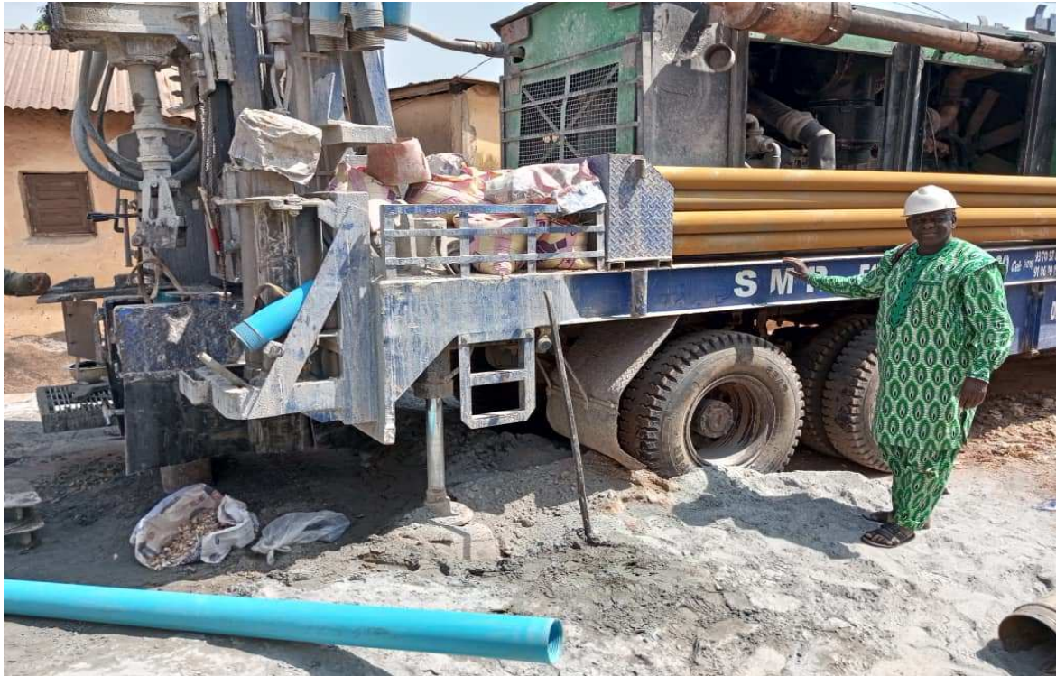
Well drilling at the Kparatao site on January 23, 2026
