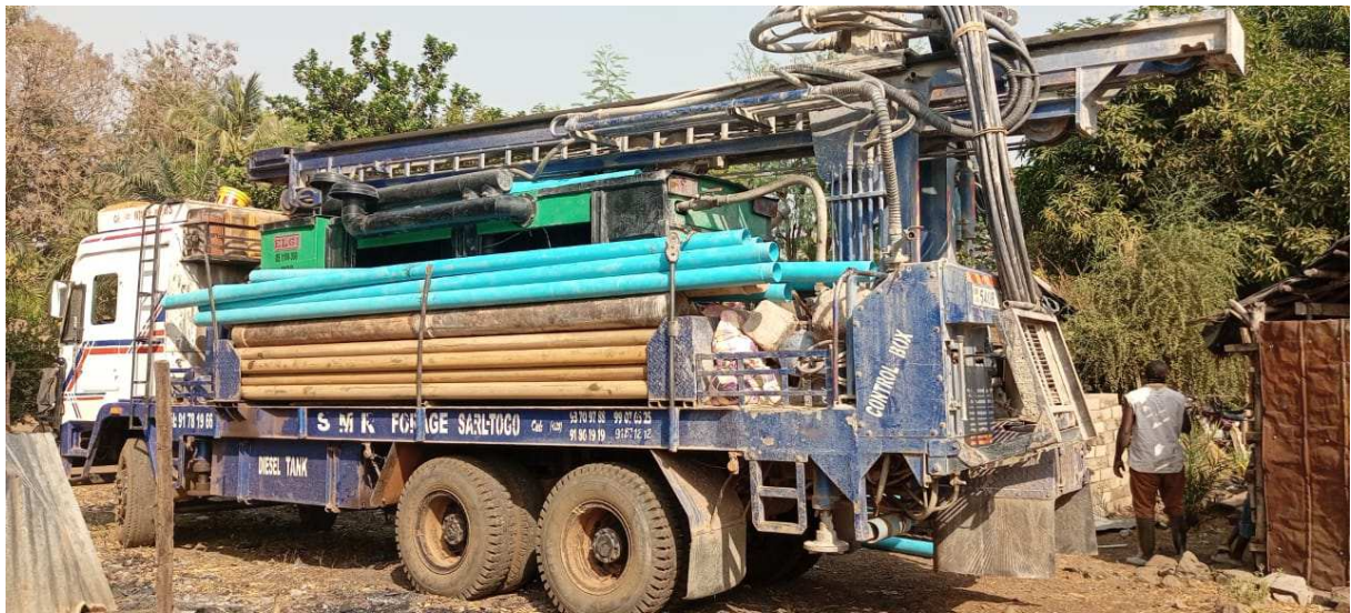
Well drilling at the Pagala -Gare canton site on January 25, 2026
