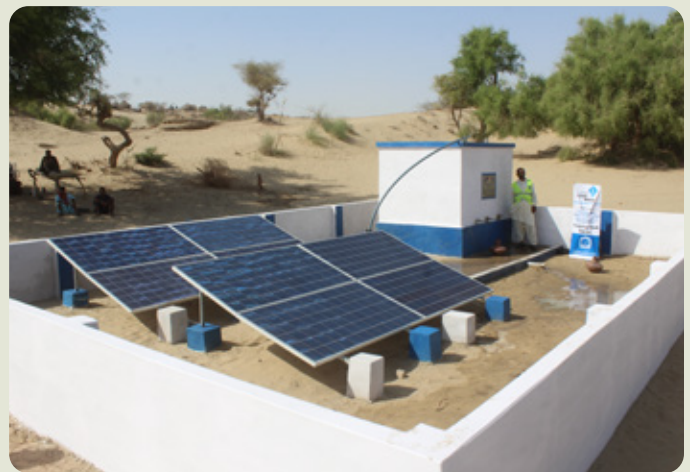
Alkhidmat installing a solar submersible water pump in Tharparkar, Sindh.
