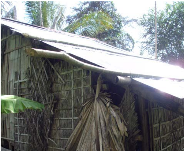
House before renovation
