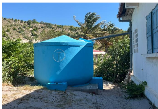
The current source of drinking water for the school and wider community of Karinoro, which is open to contaminants (left). An example of a Tatirano 10,000-litre rainwater harvesting system (right).
