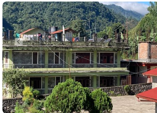
Renovation of the main building
