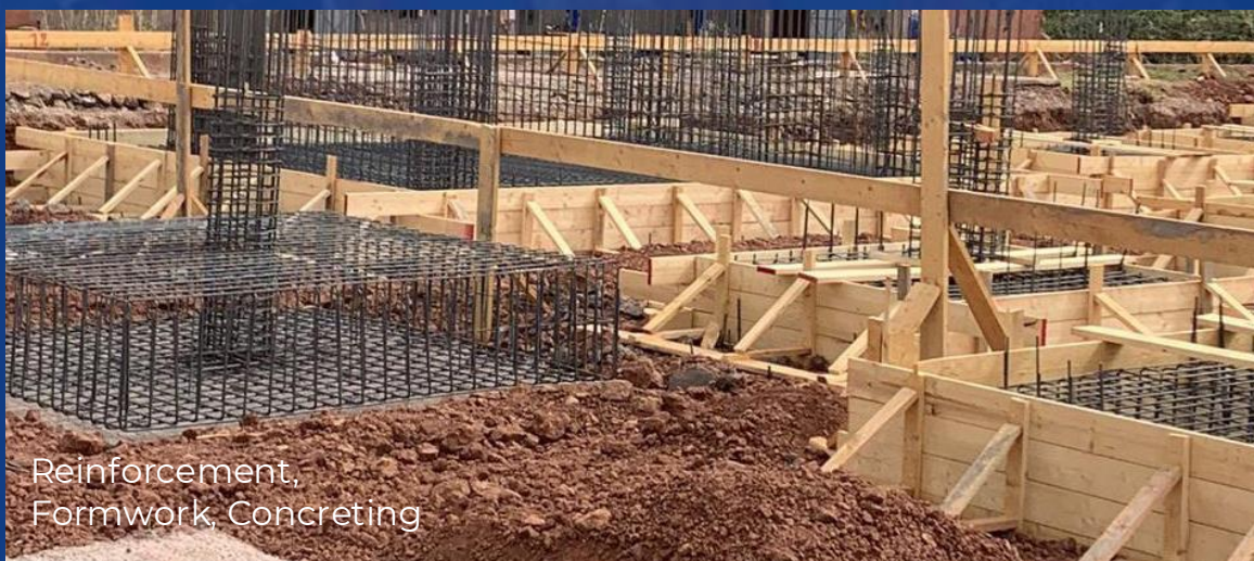
Foundation Reinforcement
