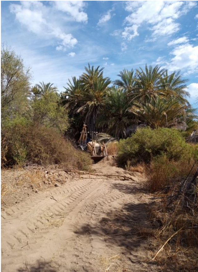
Figure 5 Machinery improving access
