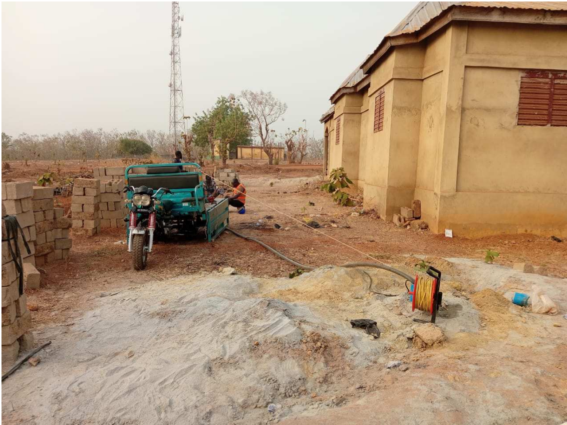
Pumping of the Kparatao Library borehole on February 8, 2025
