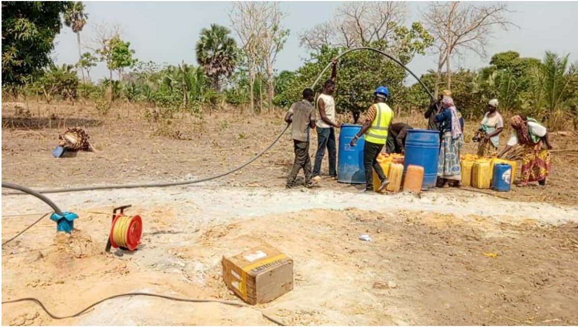
Pumping of the Tchébidè borehole on February 9, 2025
