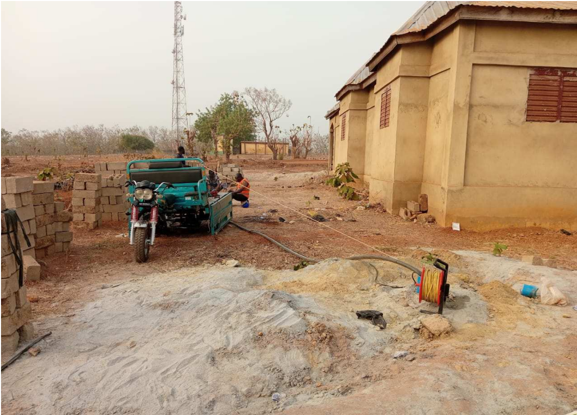
Pumping of the Kparatao Library borehole on February 8, 2025
