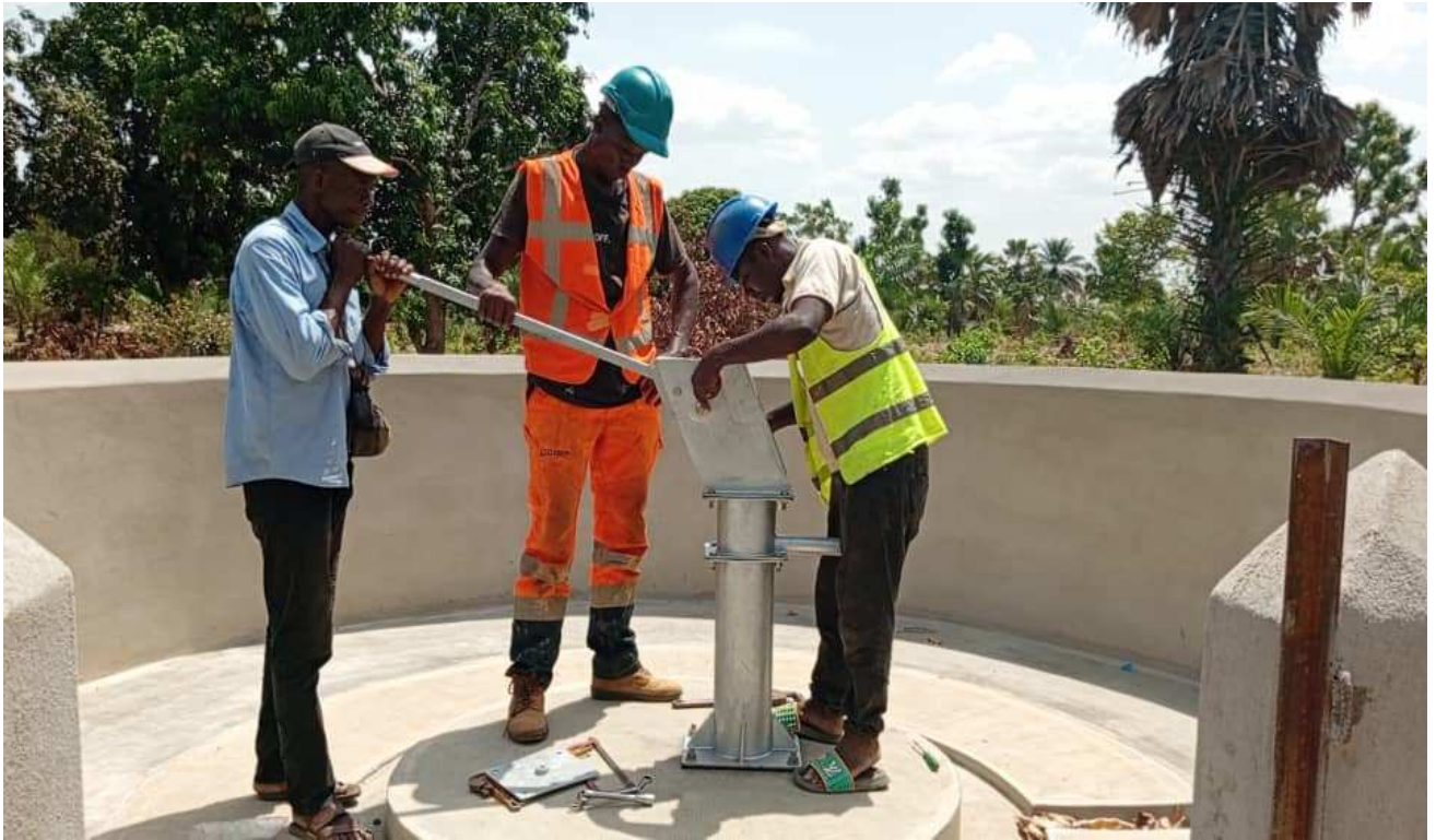
Installation of the manual pump on the Tchébidiè borehole on April 2, 2025
