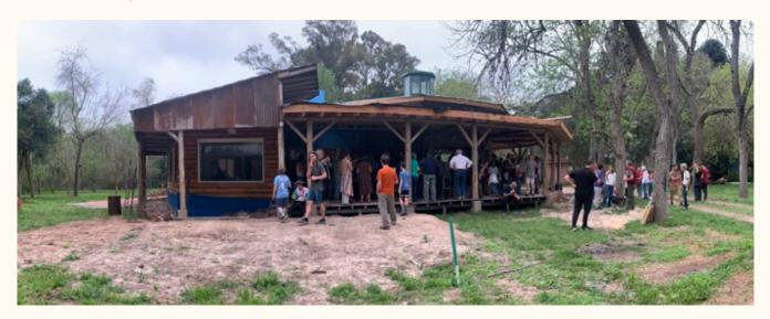
Making use of an *existing foundation*, we created a new space for events, workshops and seminars, with a large kitchen and accessible bathrooms. The sanitary spaces are brick and mortar construction and the social spaces framed with wooden logs. Ceilings are wood and concrete, with external tin and green-plant roofing.
