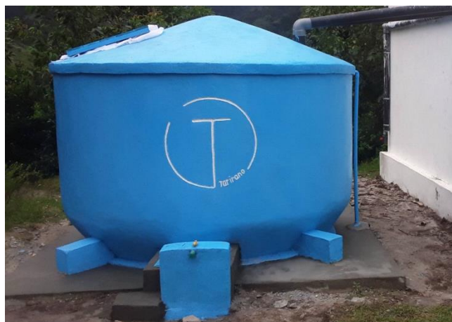
The community well in Amboavola, which is open to contaminants and in need of repairs (left). An example of a 10,000-litre rainwater harvesting system (right).
