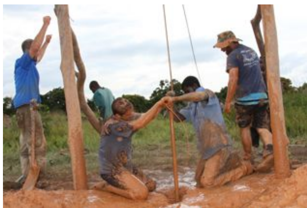
Photo: The "Baptist" drilling method developed by Water for All, International. Here it is being used by a team of local drillers in Samfya, Zambia.
