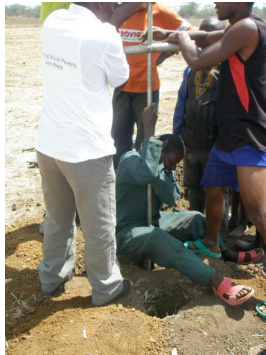
Photo: Hand-augering technique- in coordination with IDE-Zambia outside of the capital, Lusaka.
