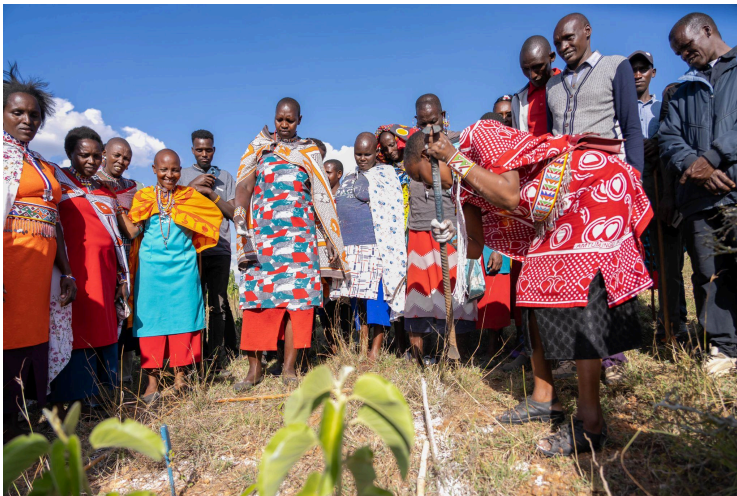
Women take lead at the official groundbreaking activity at the Eco Village
