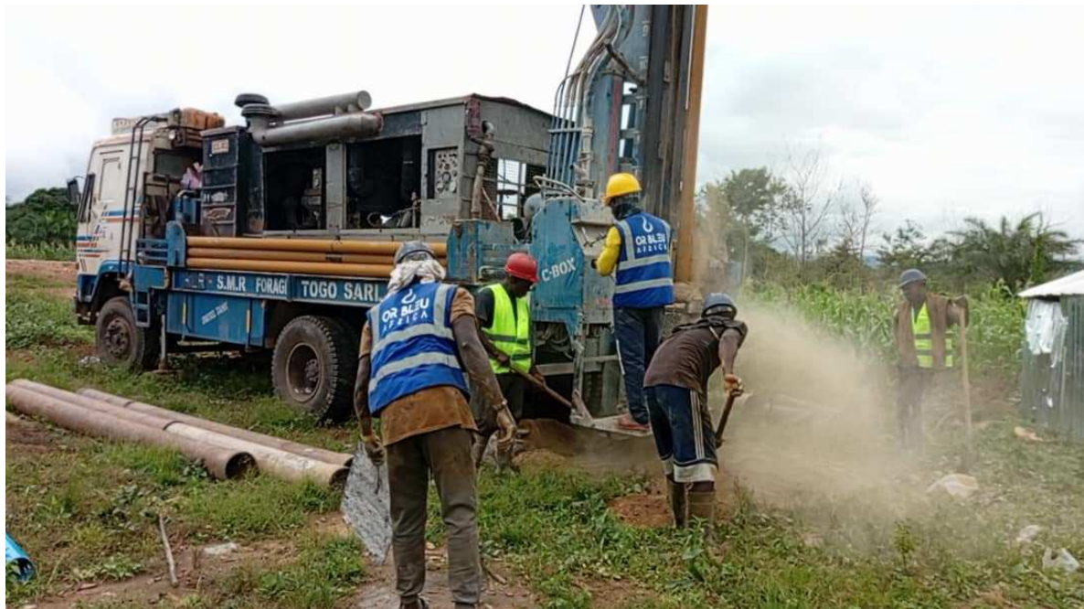
Well drilling at the project site on August 29, 2024
