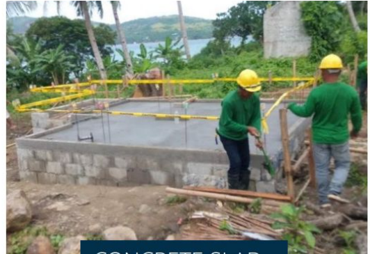
CONCRETE SLAB
