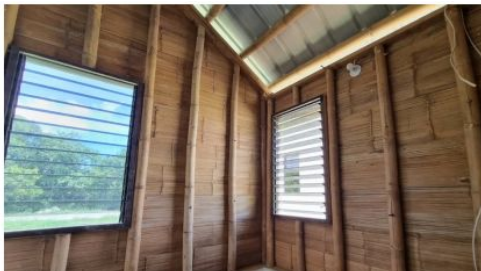
INTERIOR FINISH WITHOUT PLASTER
