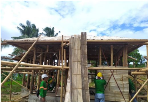
FLATTENED BAMBOO INSTALLATION
