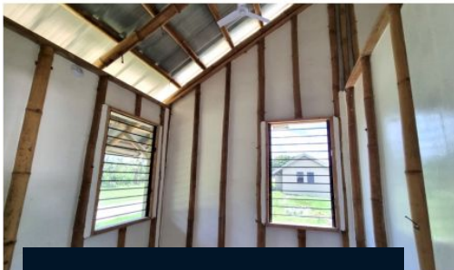
INTERIOR WITH PLASTER
