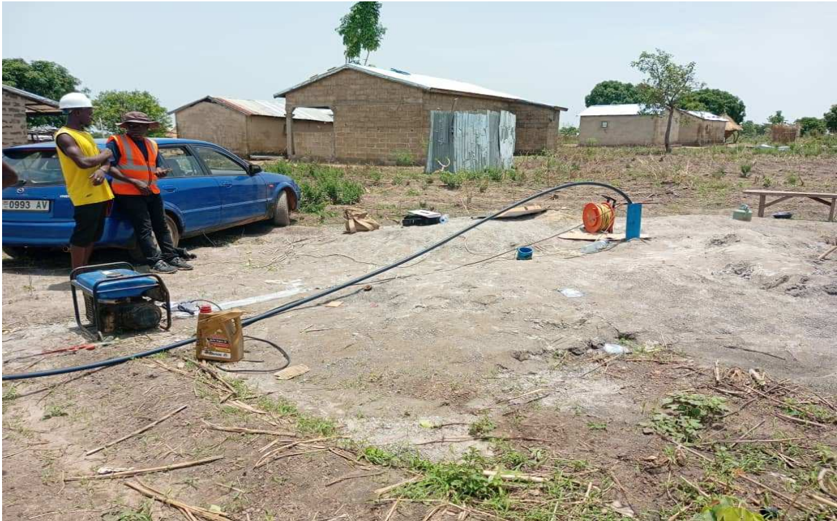
Pumping of the Lediyo / Kpalou-Kpalou borehole on April 22, 2024
