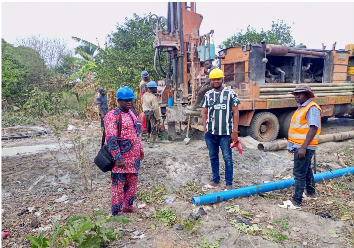
Drilling of wells on the Nigbaoudè / Darsalam site on April 9, 2024
