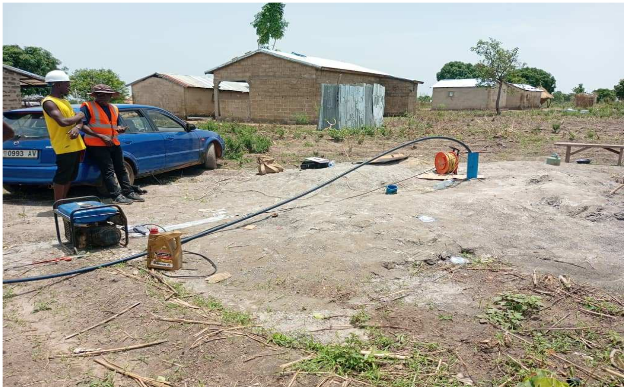
Pumping of the Lediyo / Kpalou-Kpalou borehole on April 22, 2024
