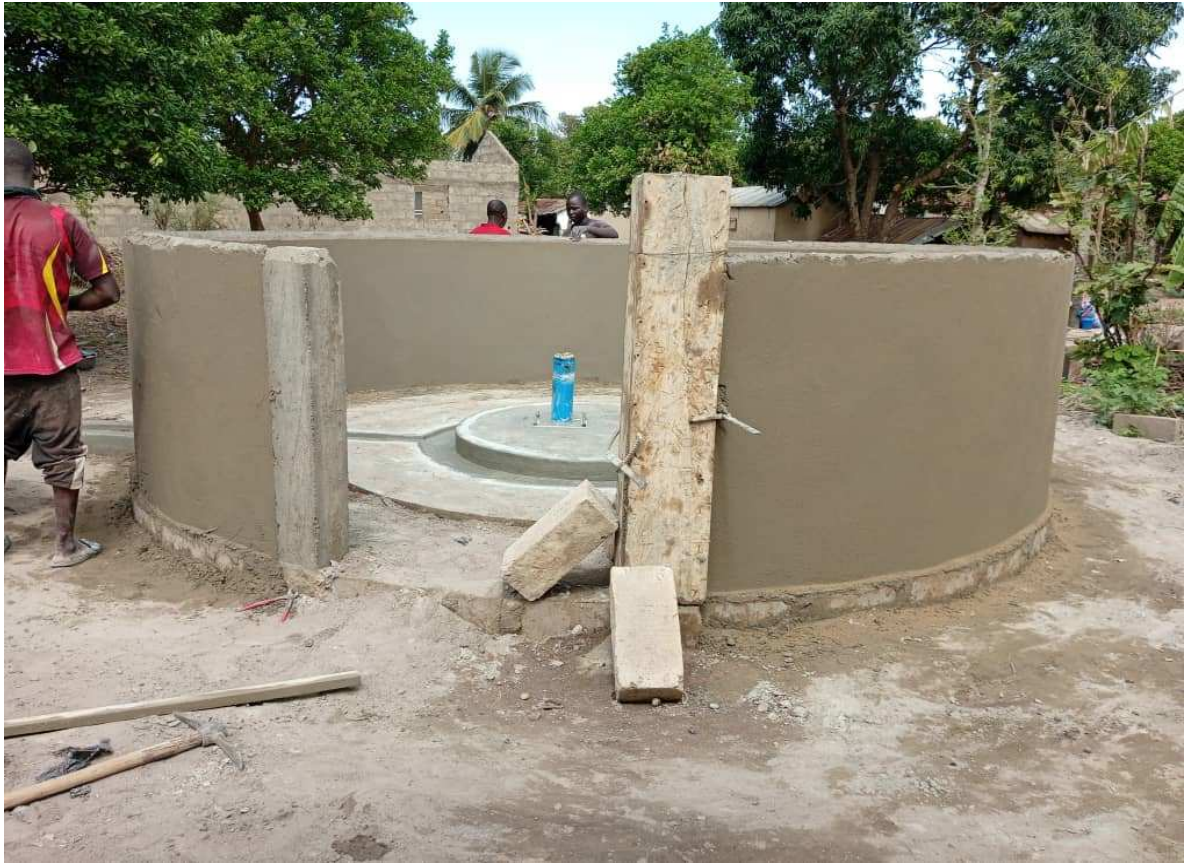
Construction of the Nigbaoudè II superstructure on May 13, 2024
