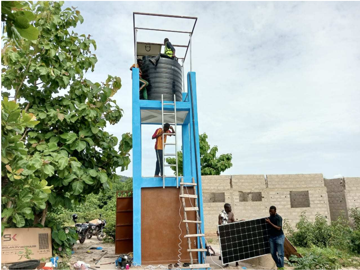
Installation of solar panels, pump and polytank on June 20, 22 and 23, 2024
