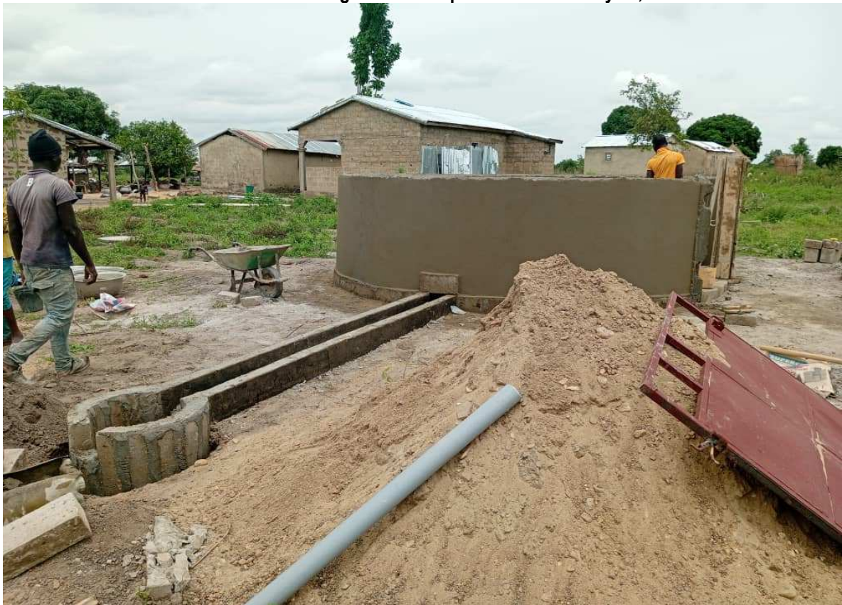
Construction of the Lediyo / Kpalou-Kpalou superstructure on May 16, 2024
