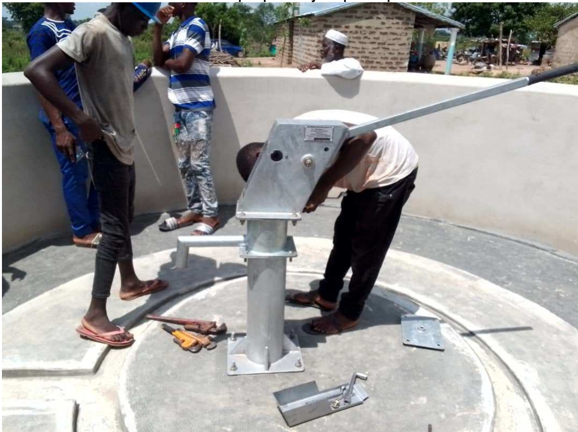
Installation of the mechanical pump in Lediyo / Kpalou-Kpalou on June 1, 2024
