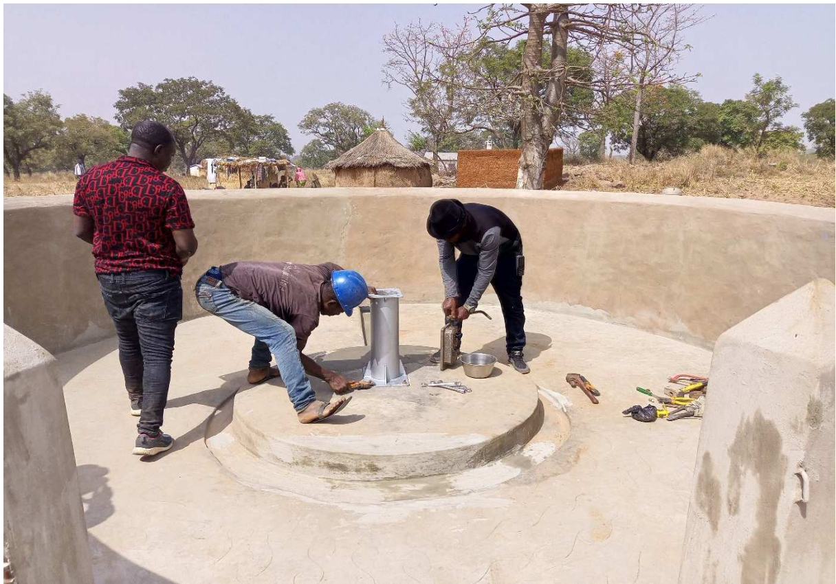
Installation of the pump on the Koudjoma II site
