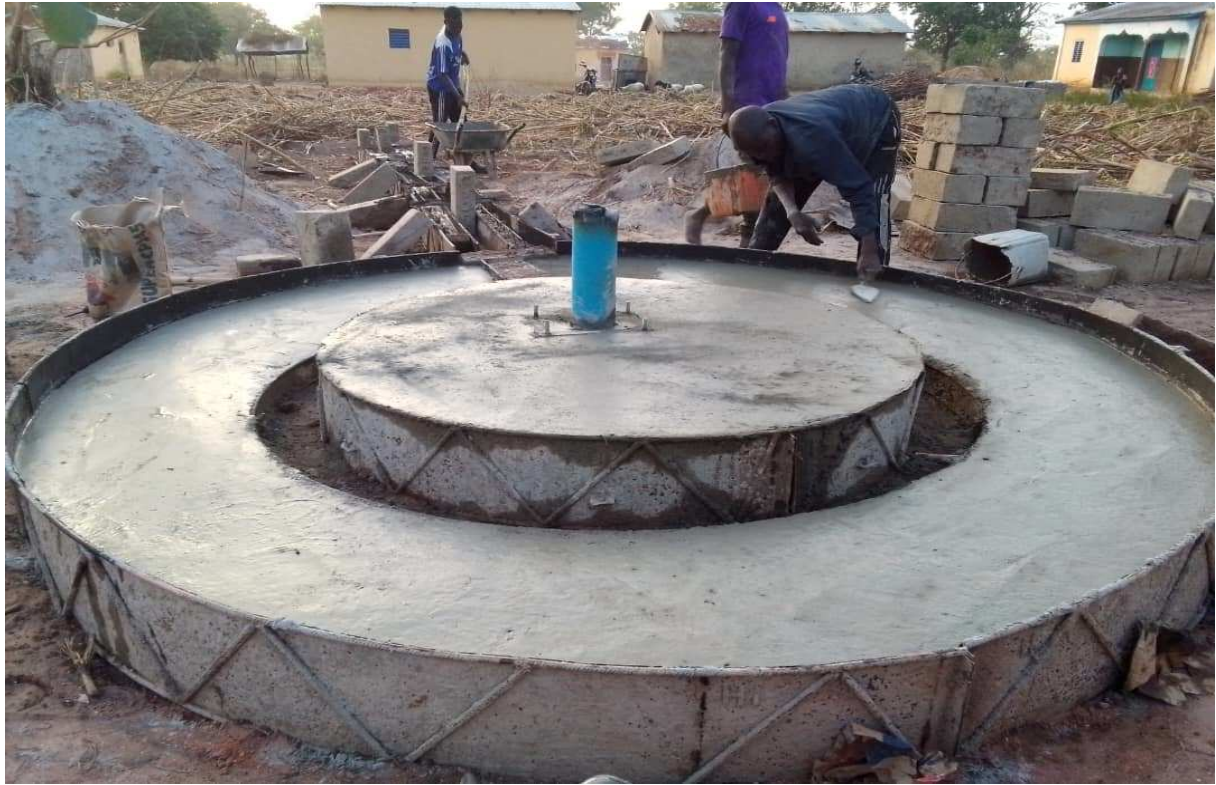
Stage of construction of the Kôbô drilling superstructure
