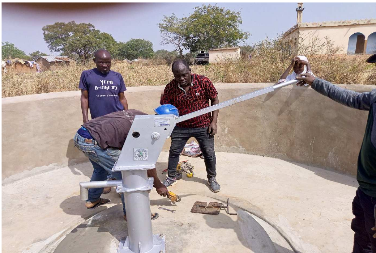
Installation of the pump on the Koudjoma II site
