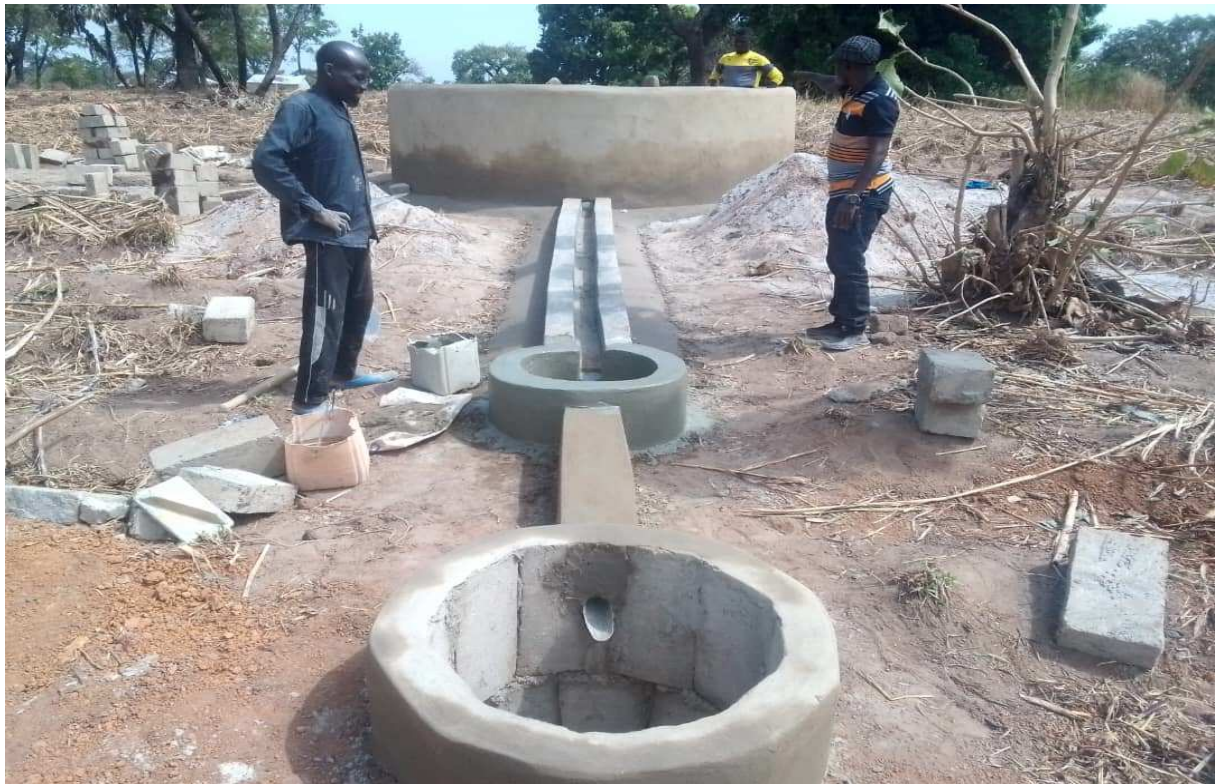
Stage of construction of the Kôbô drilling superstructure
