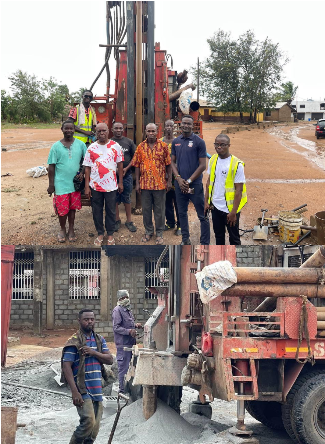
Picture Of The Ongoing Mechanized Borehole In The Achiaman Community
