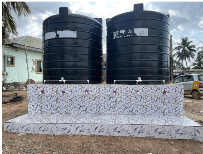
PLATFORM FULLY COMPLETED WITH THE WATER TANK
