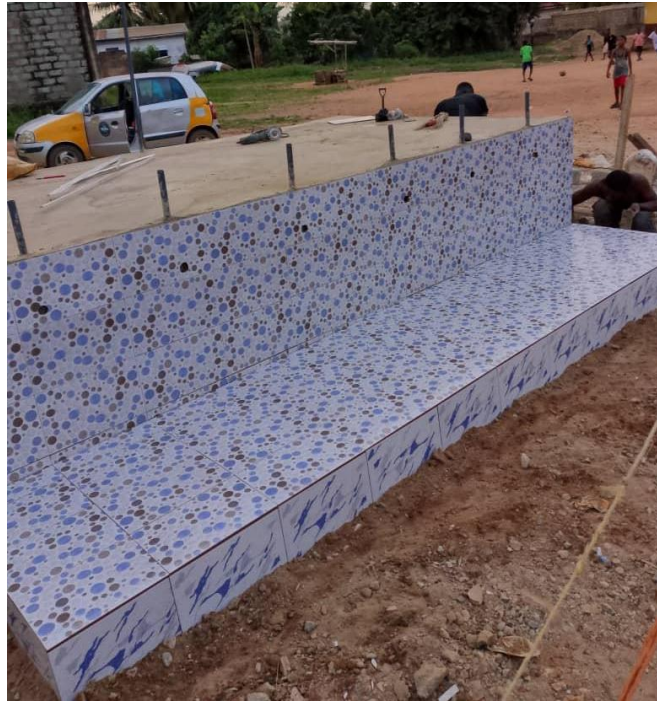
PICTURE OF THE CONSTRUCTION OF THE PLATFORM FOR THE WATER TANK
