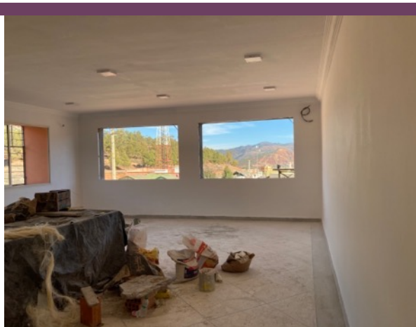
Study Centre repairs underway
