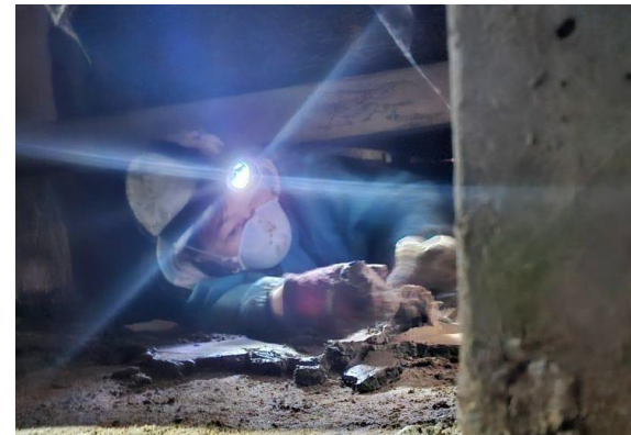
work under the floor©Vnet
