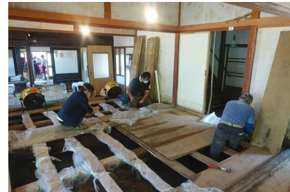
mud is being removed after curing ©Vnet
