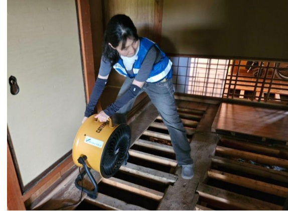
Drying work after removing mud. ©Vnet
