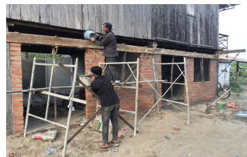
3 classrooms were built
