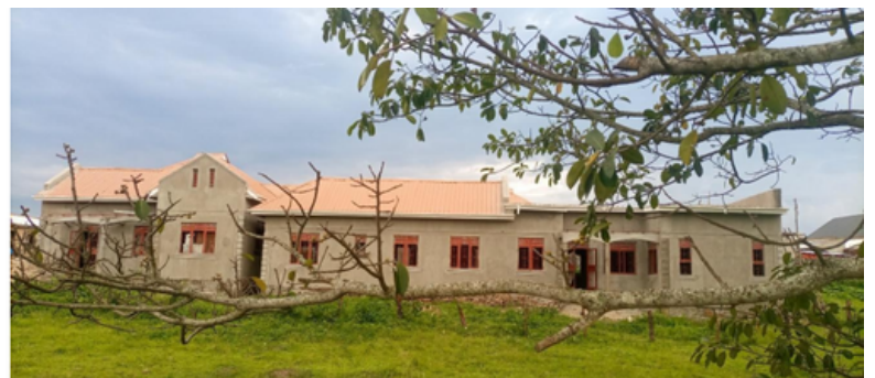
Fg.3 Replastering of the HEVIA healthcenter
