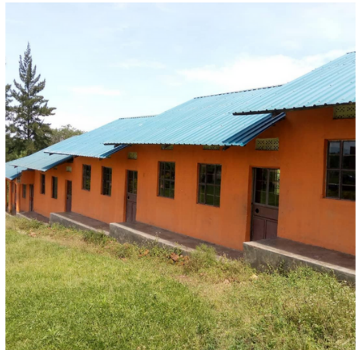
Fg.2 Repairs mad to glass windows and drainage of a partner school
