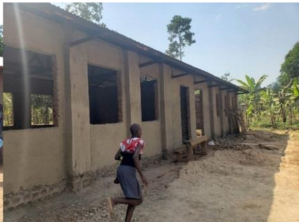
Building brick classrooms in 2022
