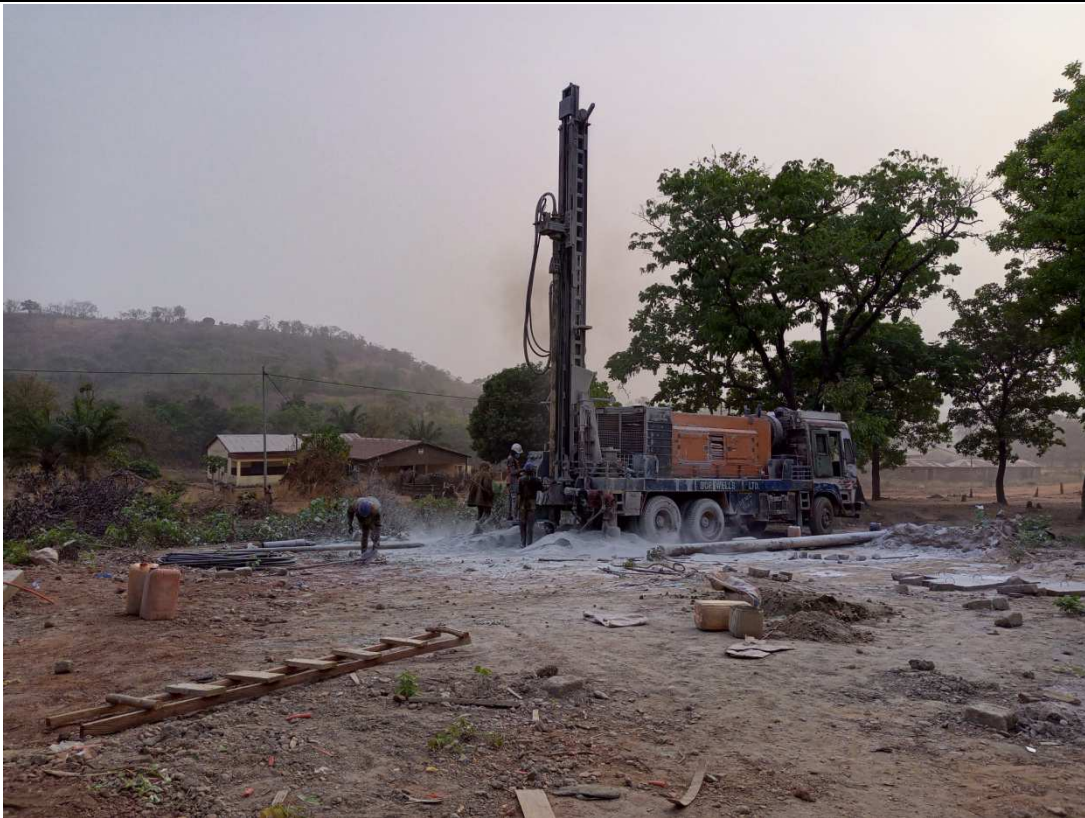
Drilling at Bowounda High School, Monday, February 20, 2023
