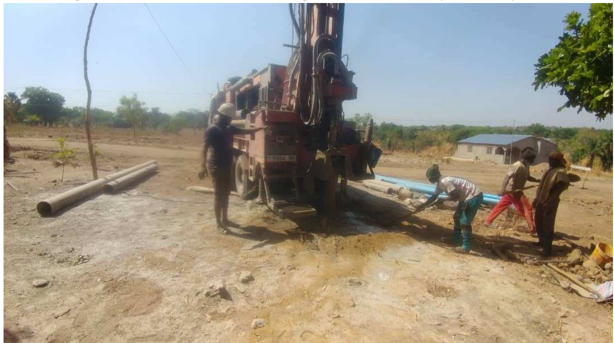
Drilling at Adam-Kôkôrô on Thursday, March 02, 2023
