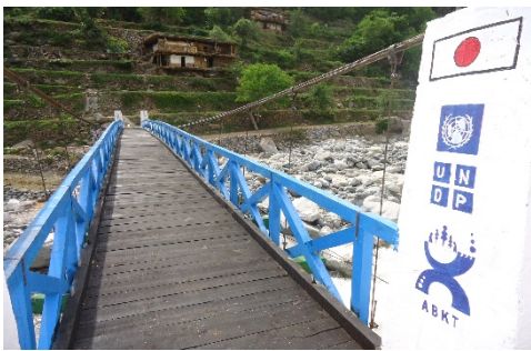
Figure 6 Suspension bridge Qashqari Upper Dir
