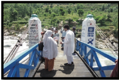
Figure 1 Suspension bridge Qolundai Upper Dir
