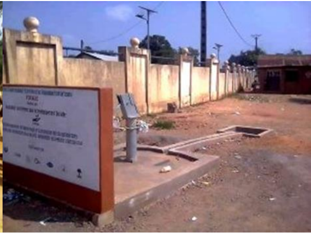
M'Poko-Bac School water borehole
