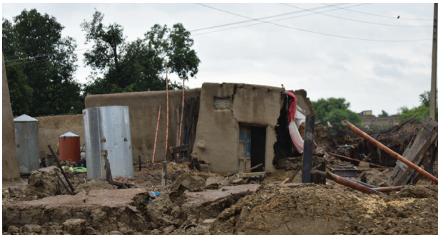
HOUSE DAMAGES HAVE FORCED SURVIVORS TO RELOCATE TO SAFER PLACES, RAJANPUR
