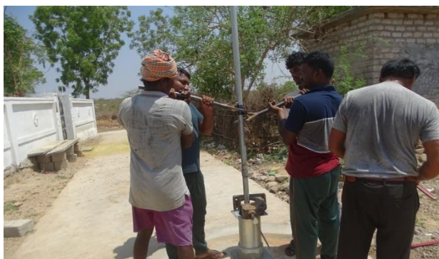
Technician &amp; village volunteers are inserting the G.I.pipes.
