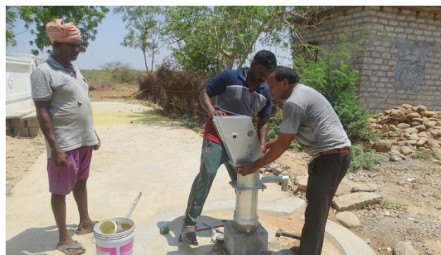
Technician and the volunteers are fixing the bore head.
