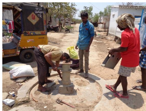
The technician removed the old head assembly, hand assembly & GI pipes for replacement.
