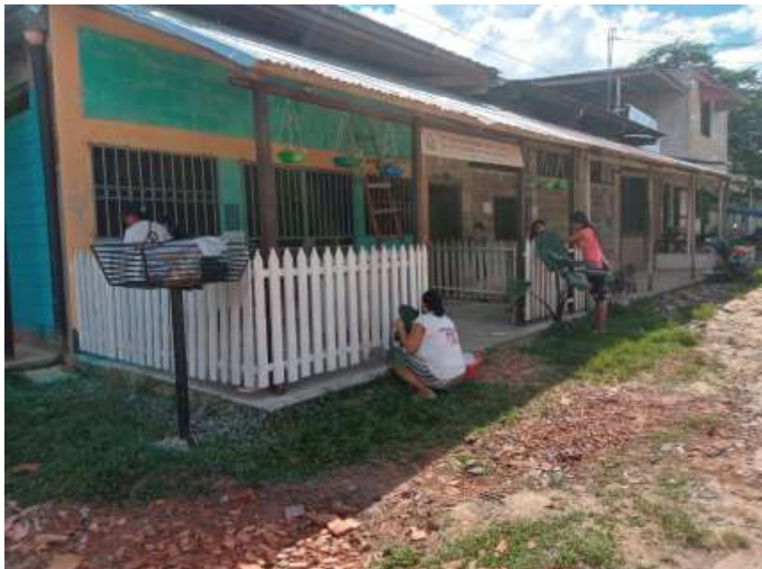
Maintenance work at Brother Policarpo Residence
