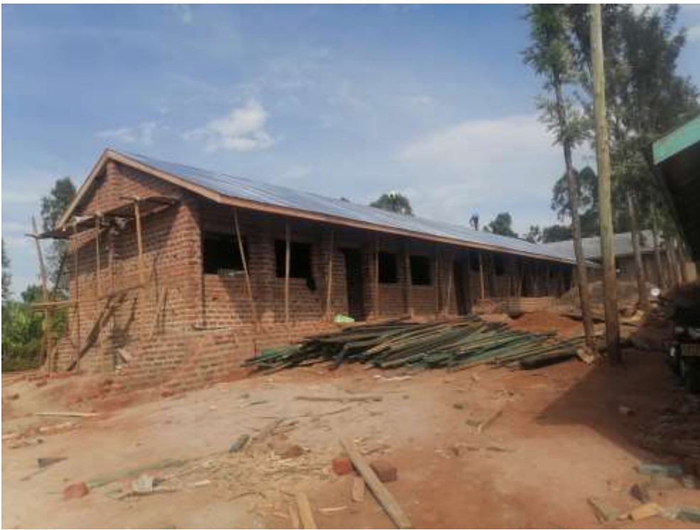
Construction work nearing completion
