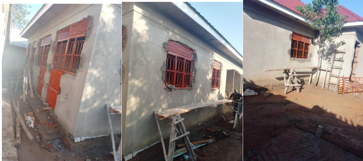
Stalled Renovation works.
